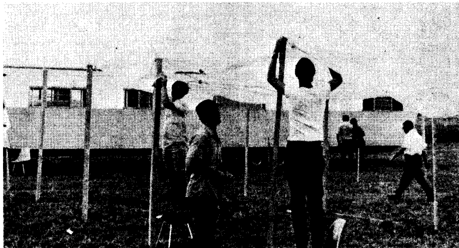
There is quite a bit of work in getting a NARAM field ready for the competition. But under the direction of the host Apollo-NASA Section and with the help of those rocketeers who arrived early and a group from Estes Industries, everything was set to go on time for the opening ceremonies.
